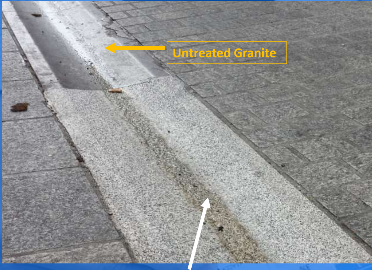
Granite drainage channel with anti-slip resin and dressing applied
